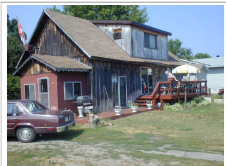
Fig 1: Dormer and deck added to the building
