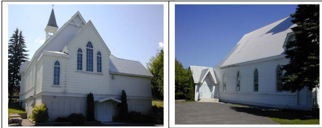
east sides of the building. Observe the door on the left side of the second photo. It is the wheelchair access and was put on the same time the basement was added to the church.
