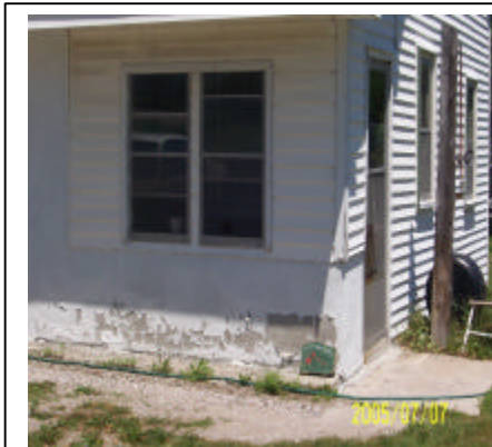
Fig 1: Original poured concrete on addition
