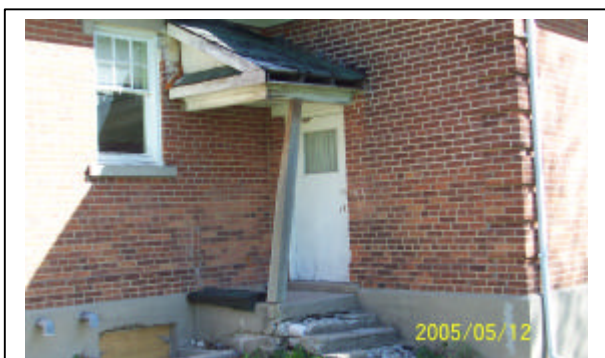
Fig 2: South side – original entrance
