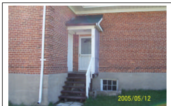
Fig 1: North side – renovated entrance
