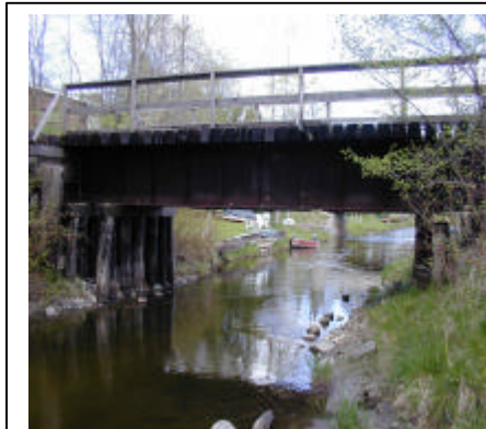
Fig 1: Log support on end of bridge and steel support beam
