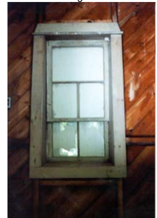
Figure 3: Window from the interior of the lighthouse.
