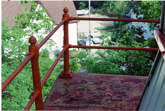
Figure 1: View of the upper deck floor and railing.
