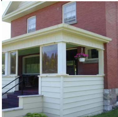
Figure 1: The enlarged veranda and porch.
