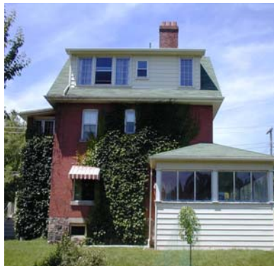
Figure 2: View of the south-east side of the house.
