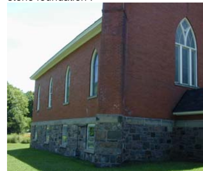
Figure 3: View of the brick walls and stone foundation.
