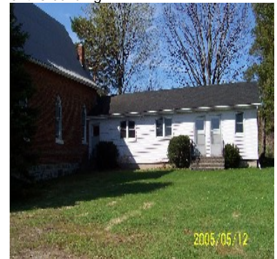
Figure 3: The 1961 addition to the side of the building.
