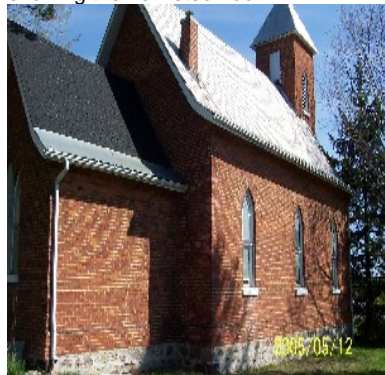
Figure 2: The roof of the church showing the new steel roof.
