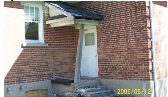
Figure 2: South side of the building with possibly the original concrete steps.
