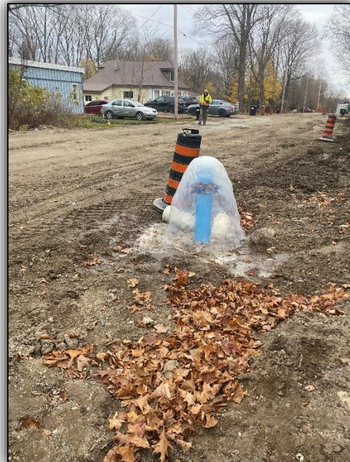
Chlorination testing using swabs on Fifth Avenue
