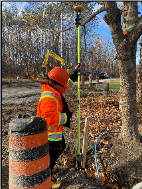
Township staff using the GPS unit for all curb stops, hydrants, and valves for our Geographic Information System (GIS) data and to create As-Built drawings.
